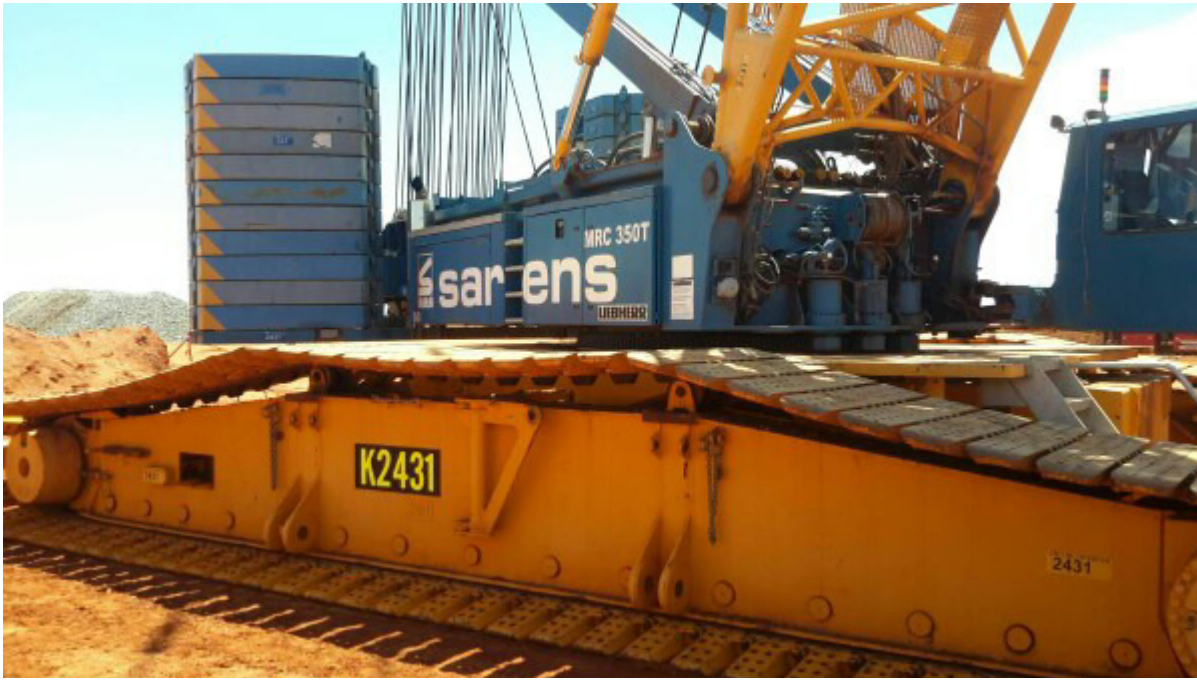
Equipment: Liebherr LR1350-1LN (2431) LOCATION: Australia
