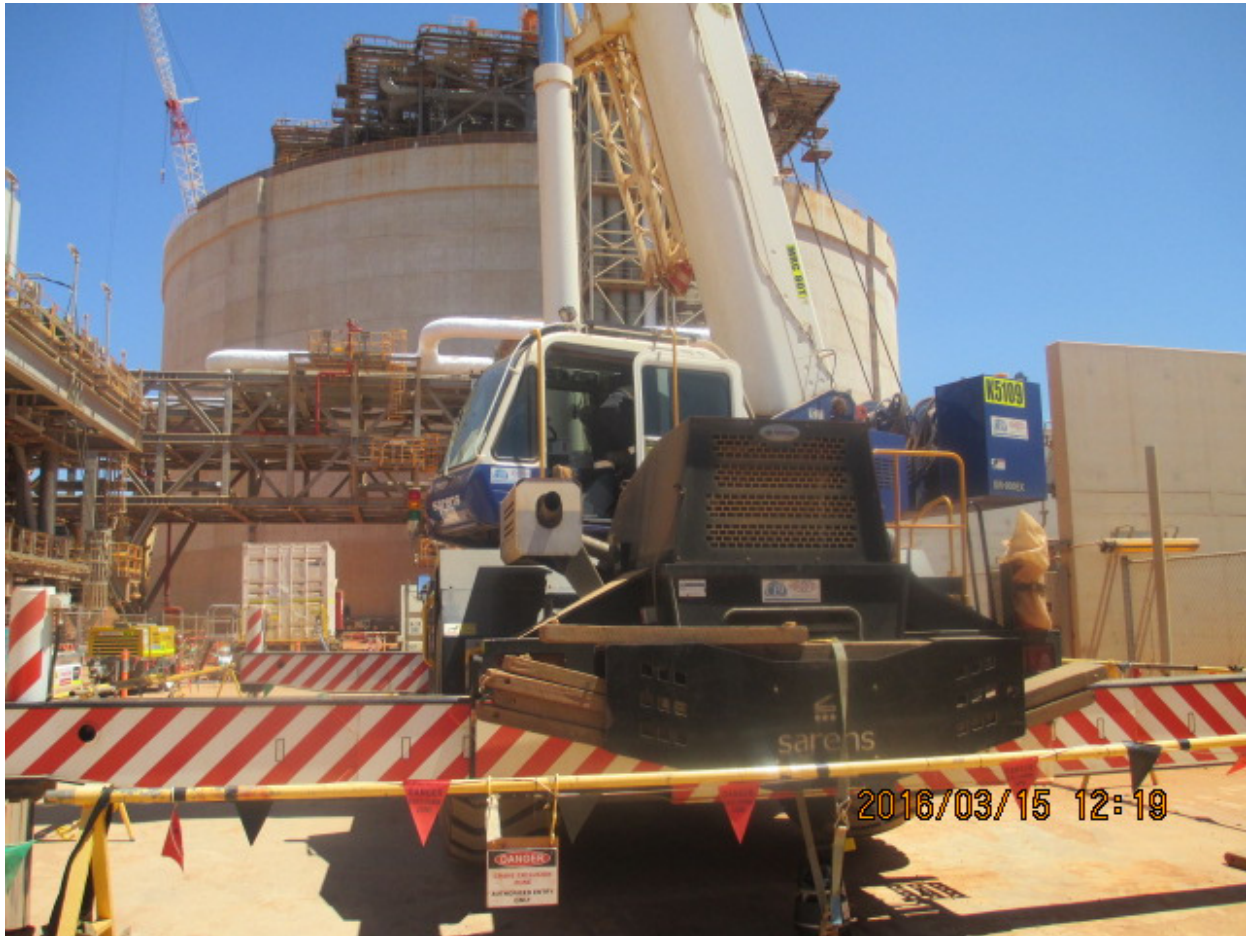
Equipment: TADANO GR800EX-2 (5109) LOCATION: WA, AUSTRALIA
