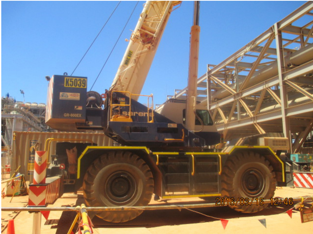
Equipment: Tadano GR800EX (5039) LOCATION: Australia
